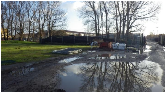
Skip and building material on site. This material stored by Welsh Water / Dwr Cymru who occupy the overall site.
