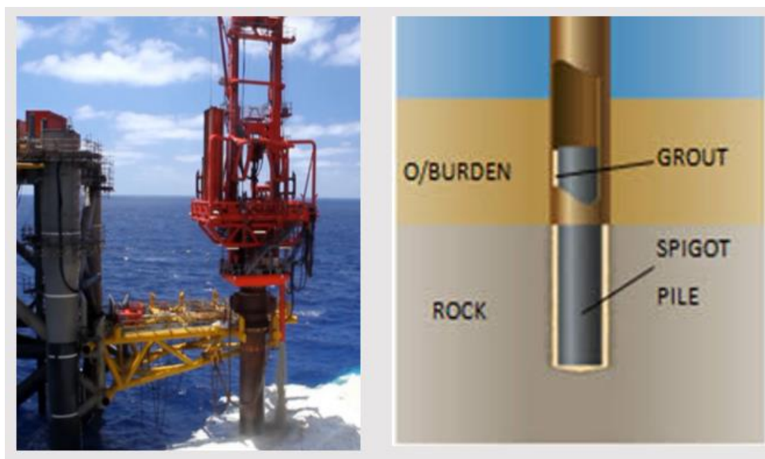
Graphic 4.10 Example of Drilled Pile (Source: OWC, 2021)
