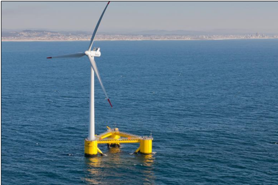
Graphic 4.3 - Example Semi-Submersible Platform, WindFloat™ Atlantic Project installed in northern Portugal. (Photo courtesy of Principle Power, Artist: DOCK90)
