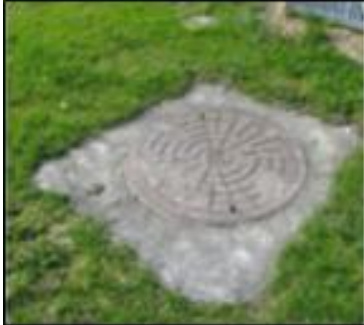
Graphic 4.17 – Earth link boxes surface and above ground
