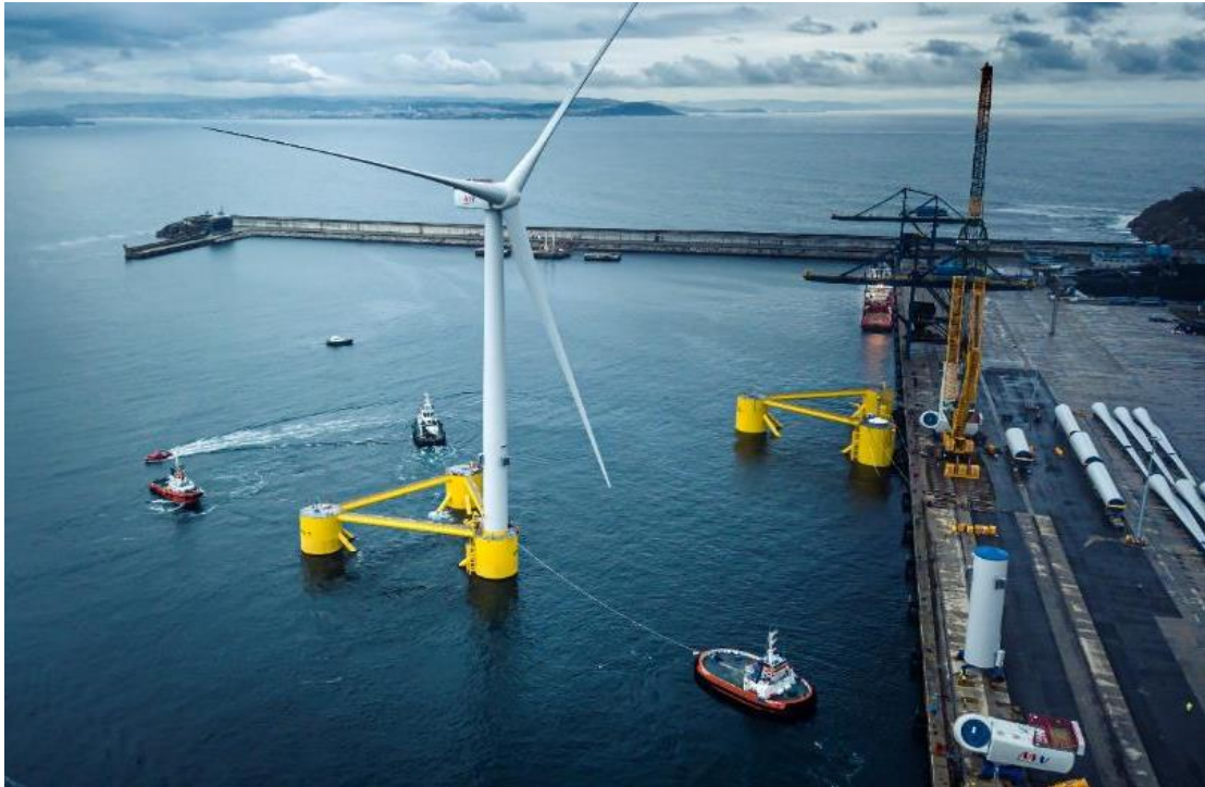
Graphic 4.19 – Example of Assembly of Wind Turbine Generator onto a WindFloat™ Platform at Quayside and Towing Out (Source: Photo courtesy of Principle Power. Artist: DOCK90)
