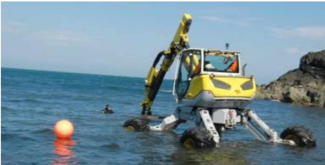
Graphic 4.22 – Menzi Muck Spider Excavator (Source: Nexans, 2021)
