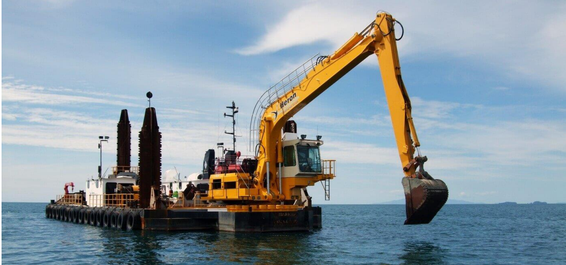
Graphic 4.21– Barge-Mounted Backhoe Excavator (Source: Courtesy of Seatools, 2021)
