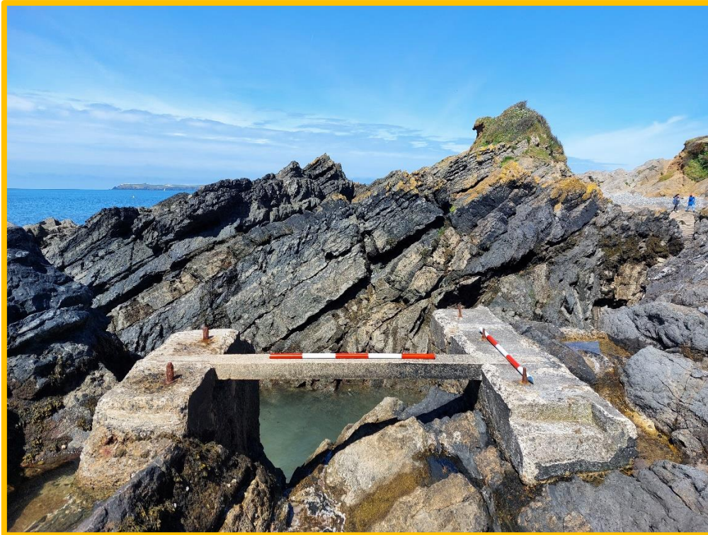
Figure 43 Possible crane base (MSDS_Erebus_309)
