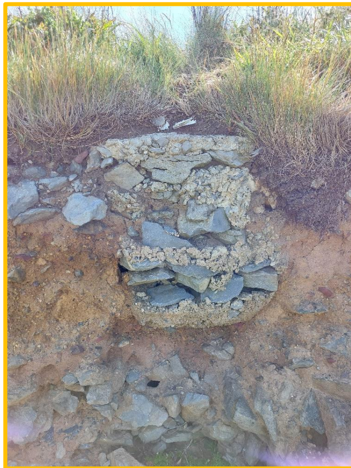
Figure 42 Concrete post (MSDS_Erebus_307)
