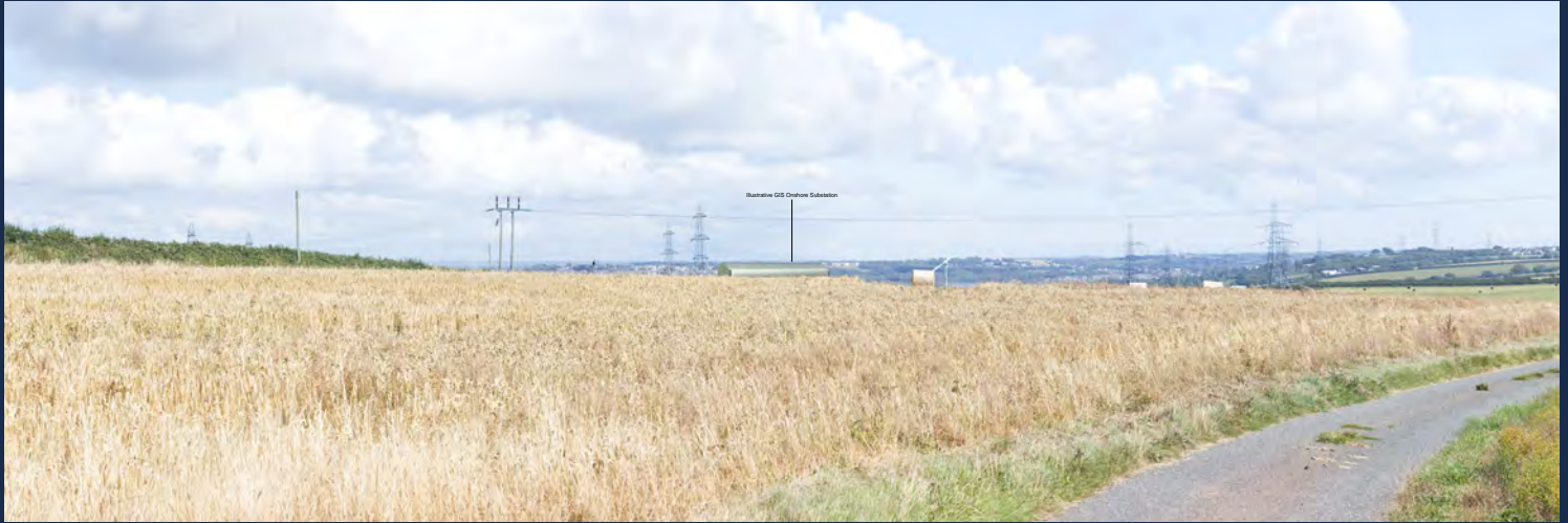
Indicative View of Substation viewed from Goldborough Road east of Wallaston Cross at year 1 (with no planting mitigation)
