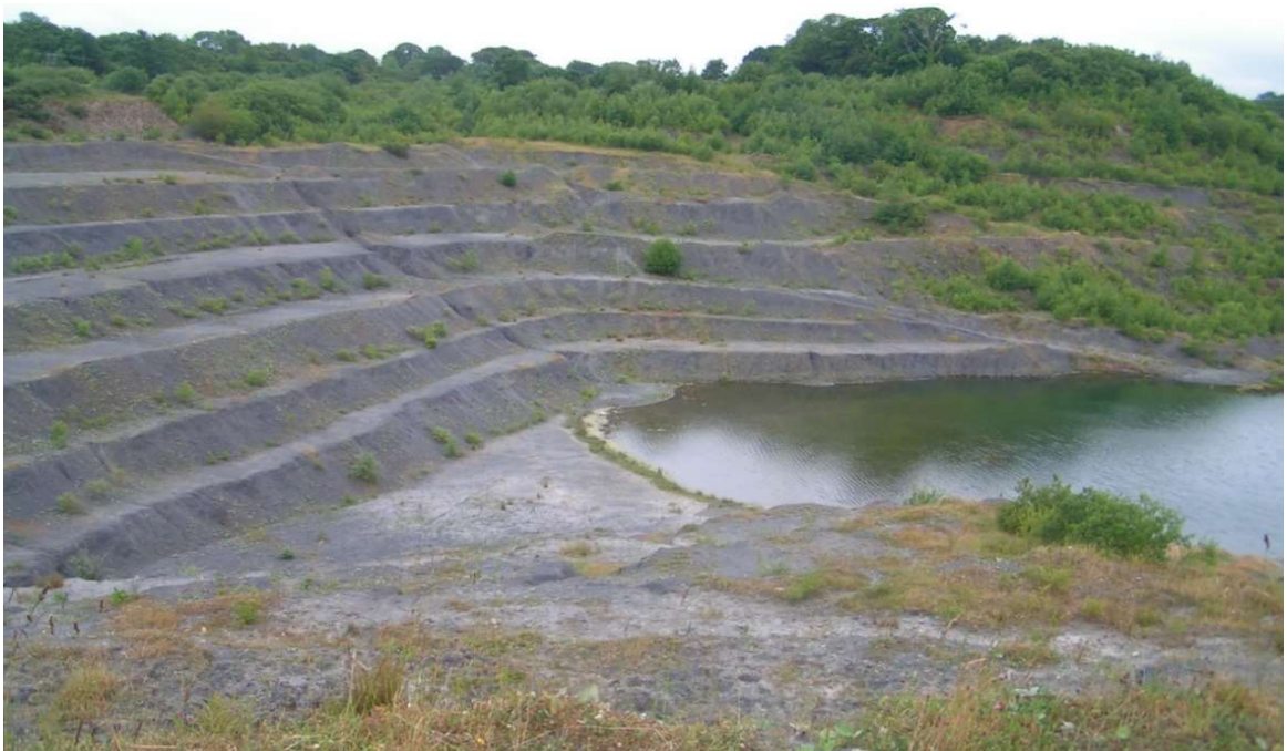
Figure 4.1: 10-year-old benches in the south face of the quarry. The foreground vegetation is a mix of annual and perennial herbaceous plants growing on bare, weathered overburden, while growth on the benches (left) only occurs in accumulated wash-off from the steep slopes. The background slopes to the
