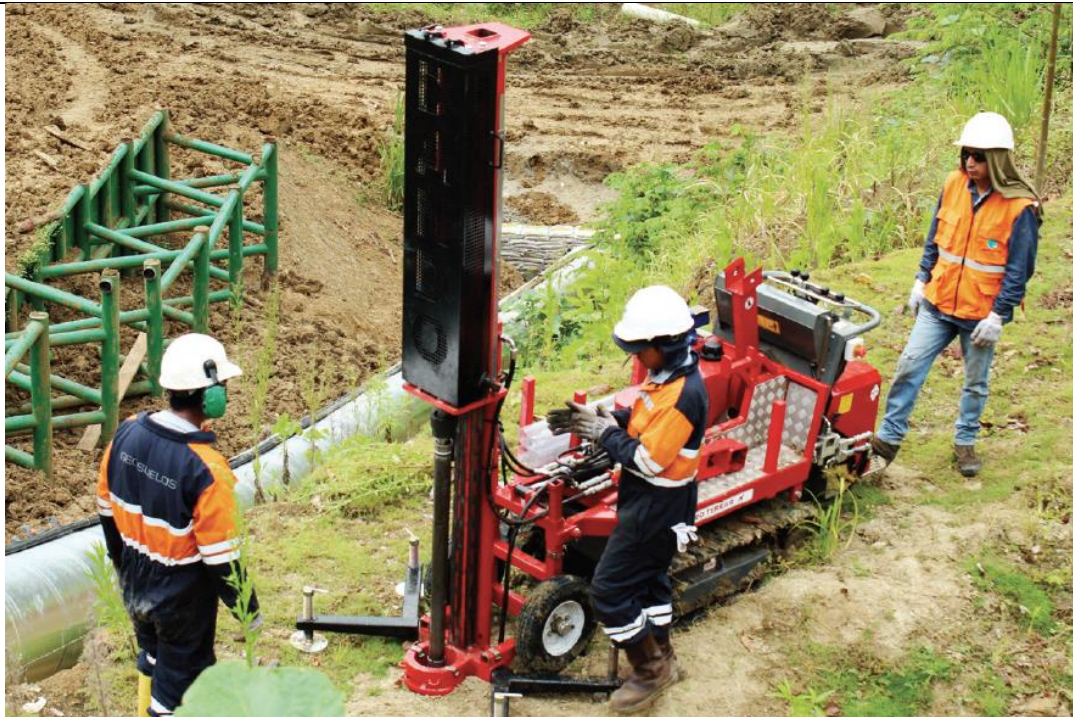
Terrier Rig tracked boring rig
