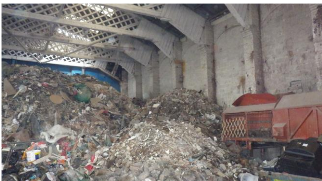
Hardcore stored in front of the trommel preventing access to it
