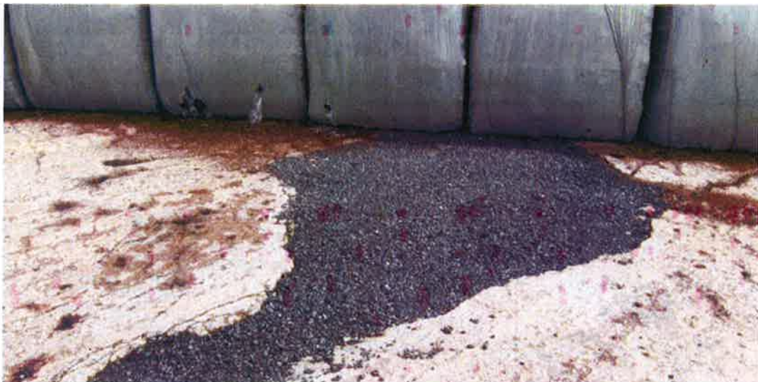
Photograph 3.2: Damage to the tertiary containment surfaces
