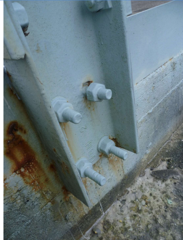
b) Support posts retained by four bolts which may need to be removed.
