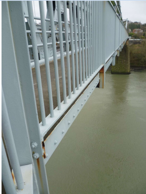
a) Railing support posts bolted onto metal support joist on the parapet.
