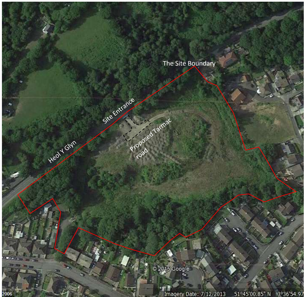
Figure 1: The Proposed tarmac road within the Heol Y Glyn site to prevent debris runoff onto the Heol Y Glyn road.
