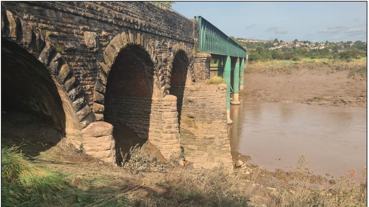
Figure 2: St Julian's Viaduct (Southern Shore – receding tide).
