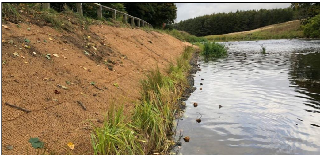
Figure 9: CocoBN used to stabilise embankment.
