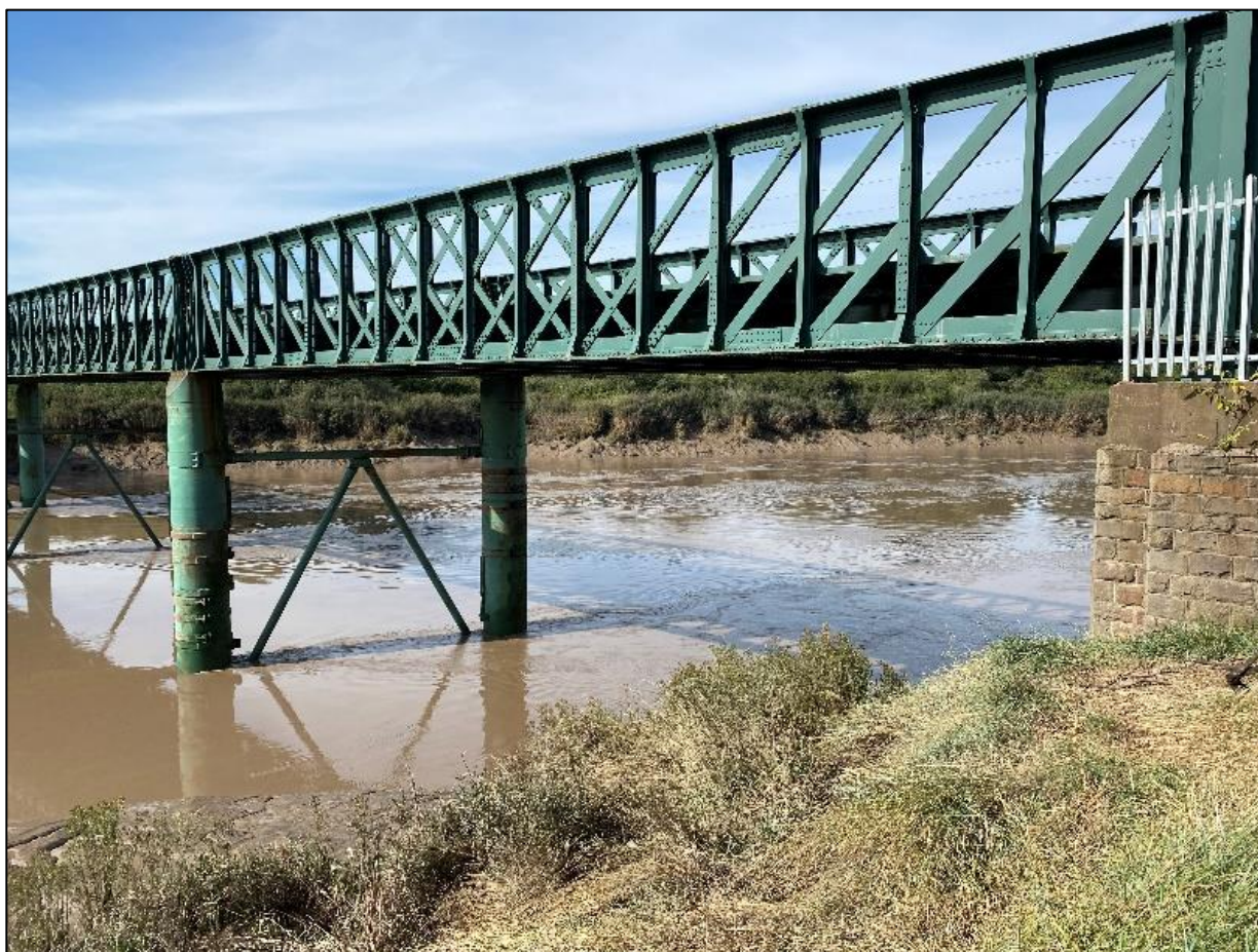
Figure 3: Saltmarsh extent to northern access
