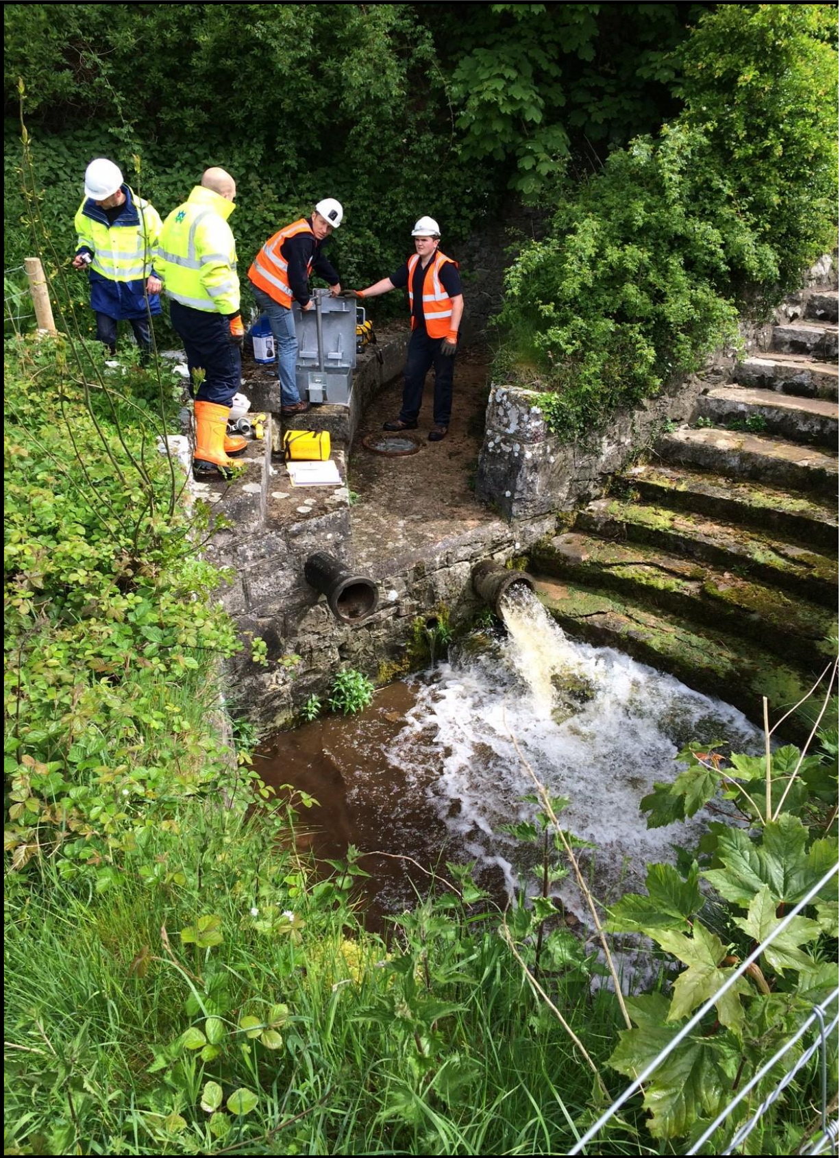
Figure 3 -Flow coming from low level outlet/ washout
