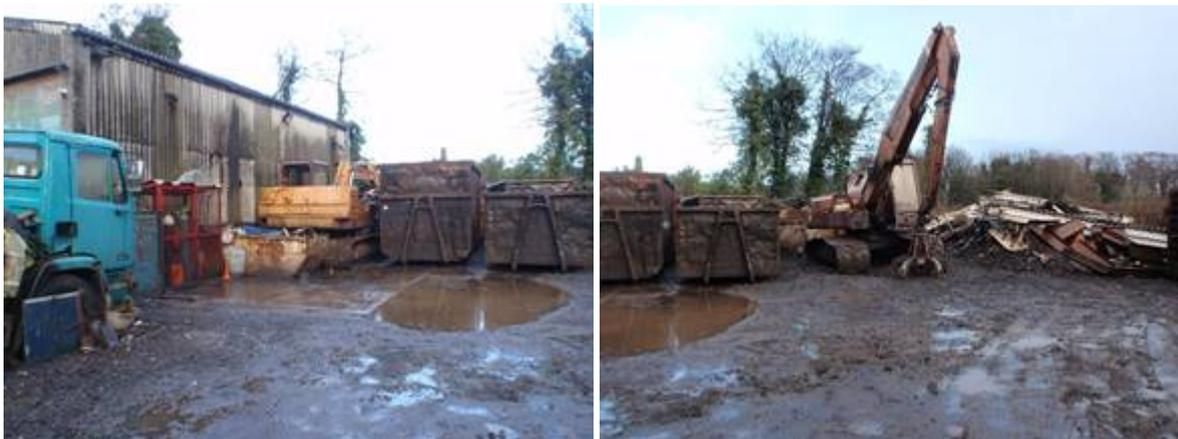
Impermeable pavement had been installed, yet no sump has been installed to serve the impermeable pavement as required under Table 2.3 – Operating Techniques of SR2011No2 and SR2011 No3. The impermeable pavement does not fully comply with the requirements of Table 2.3 as the impermeable pavement is currently not connected to a sealed drainage system, either a sealed sump or to public sewer.
