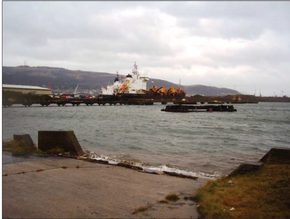
Plate 3 Queens dock view north from western end(14 th January 2013)
