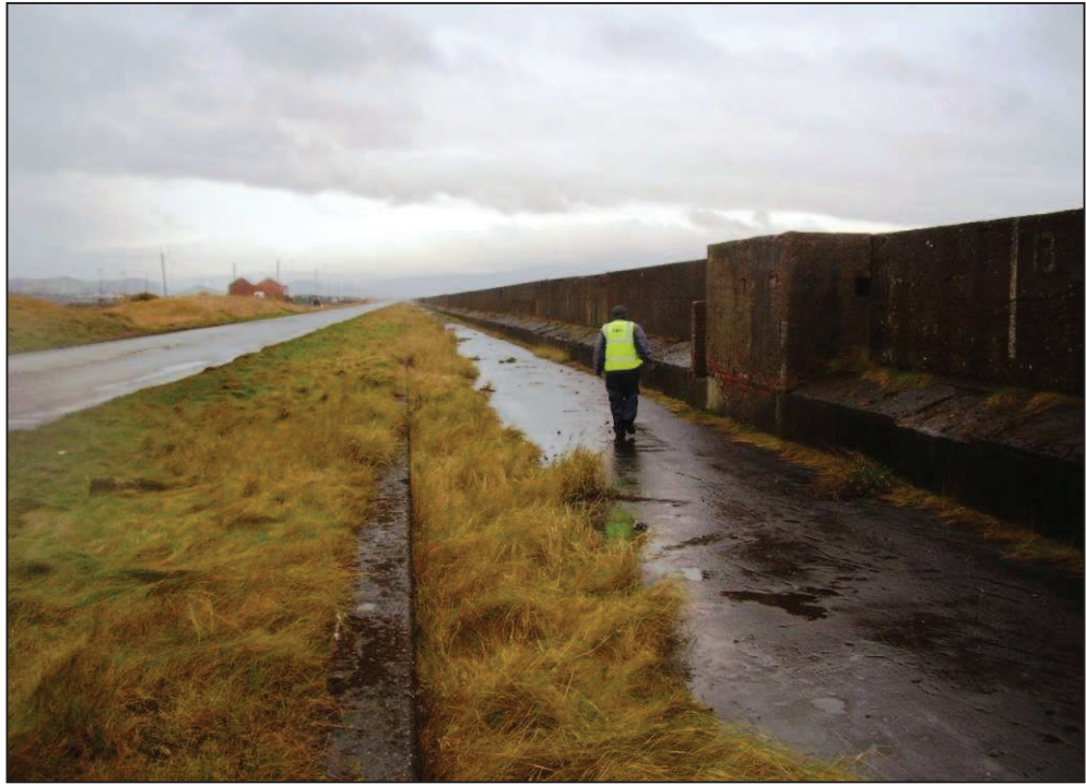
Plate 5 Sea wall with Pill box 270418 (Q2), Queens Dock to left(14 th January 2013)
