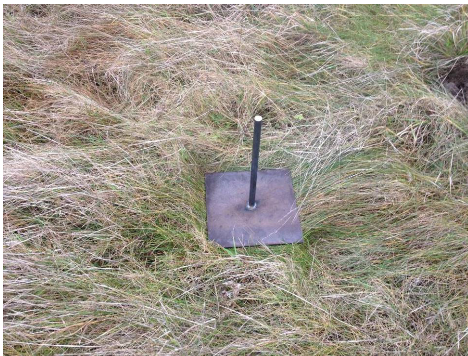
Plate 5-1 Permanent Settlement Marker on MCL (Before Final Installation)
