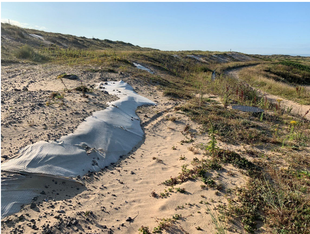
Plate 2-3 Exposed geomembranes on southwestern flank
