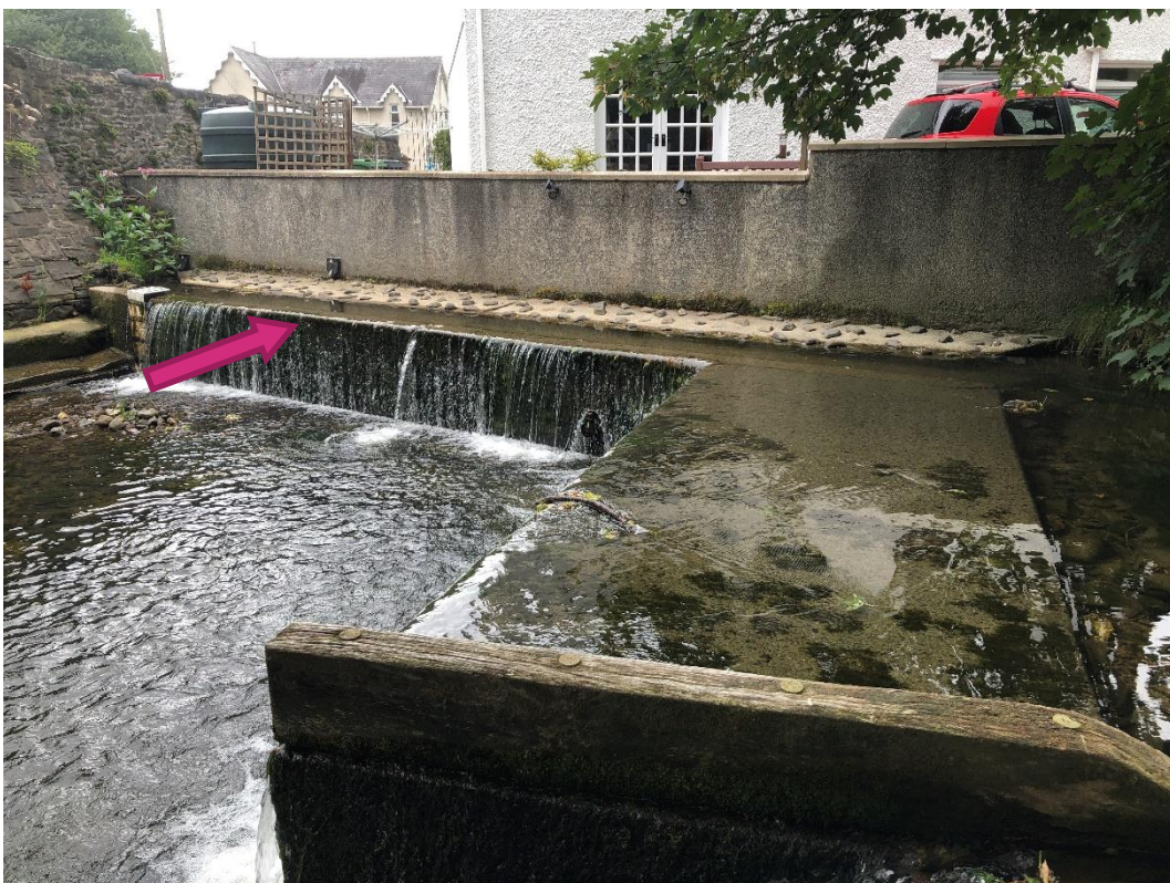
Figure 9: Leat coming off from Weir, wooden edge of low flow channel also shown. (Arup, 2020)
