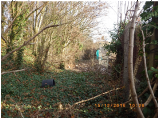
Repaired perimeter fence
