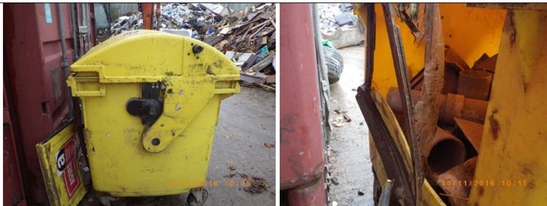
Quarantine (Asbestos) skip that was not sealed and un-bagged asbestos visible inside
