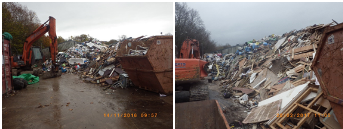
Comparison of waste on site between 14/11/2016 and 20/02/2017
