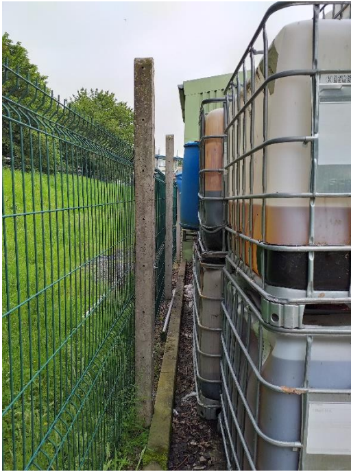
Lack of spacing between container storage and fencing adjacent to warehouse. Blue drum leaning on fence.
