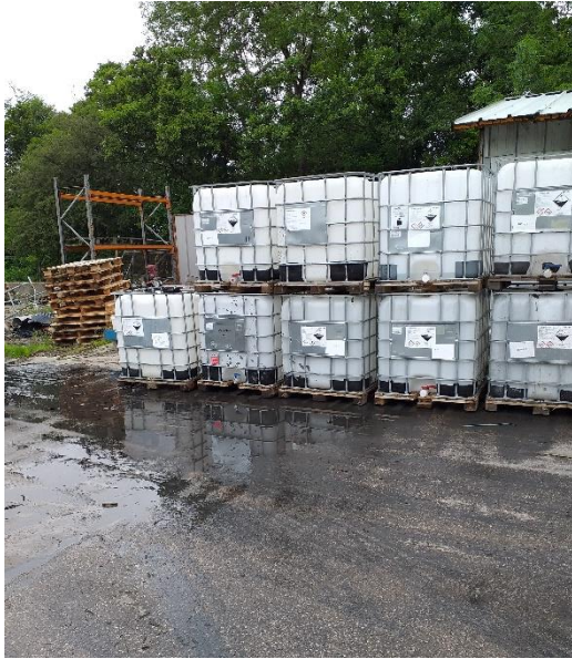
Formic acid containers stored adjacent to area of permeable surfacing
