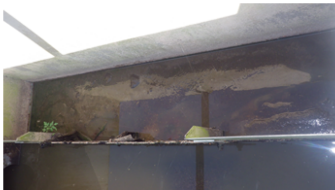
Photo showing the storm weir with damaged seal
