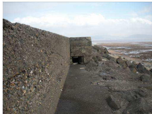
Plate 2: Pill box window allowing potential access through the sea wall for Otters (taken 11/04/2013).
