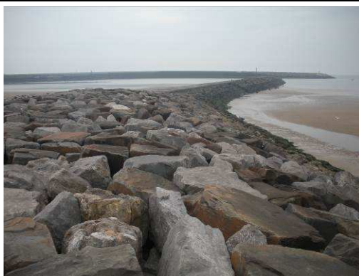
Plate 13: Rock armoured sea wall at Aberafan (photos taken 23/08/2013)
