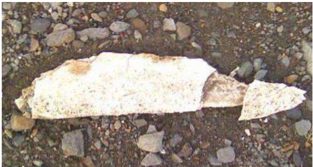
Photograph 18.5 Fragment of cladding debris collected for analysis (7 February 2013).
