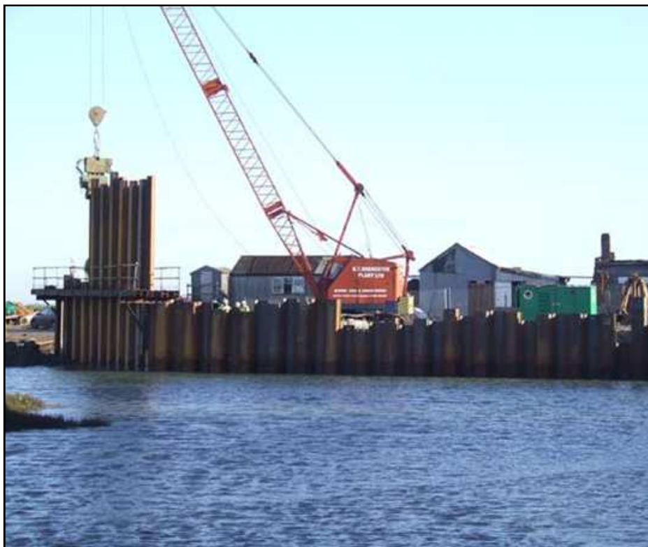
Figure 4.55 Installing sheet piles harbour side
