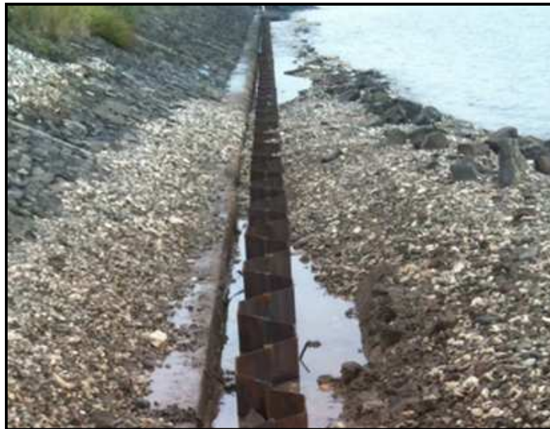
Figure 4.14 Sheet pile wall
