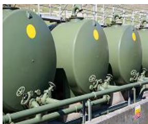
Storage tanks inside a concrete bund.
