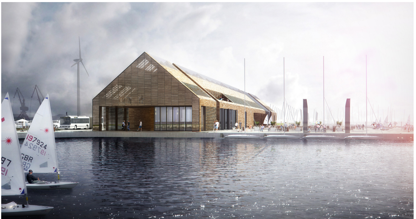
Figure 10: Western Landfall Building
