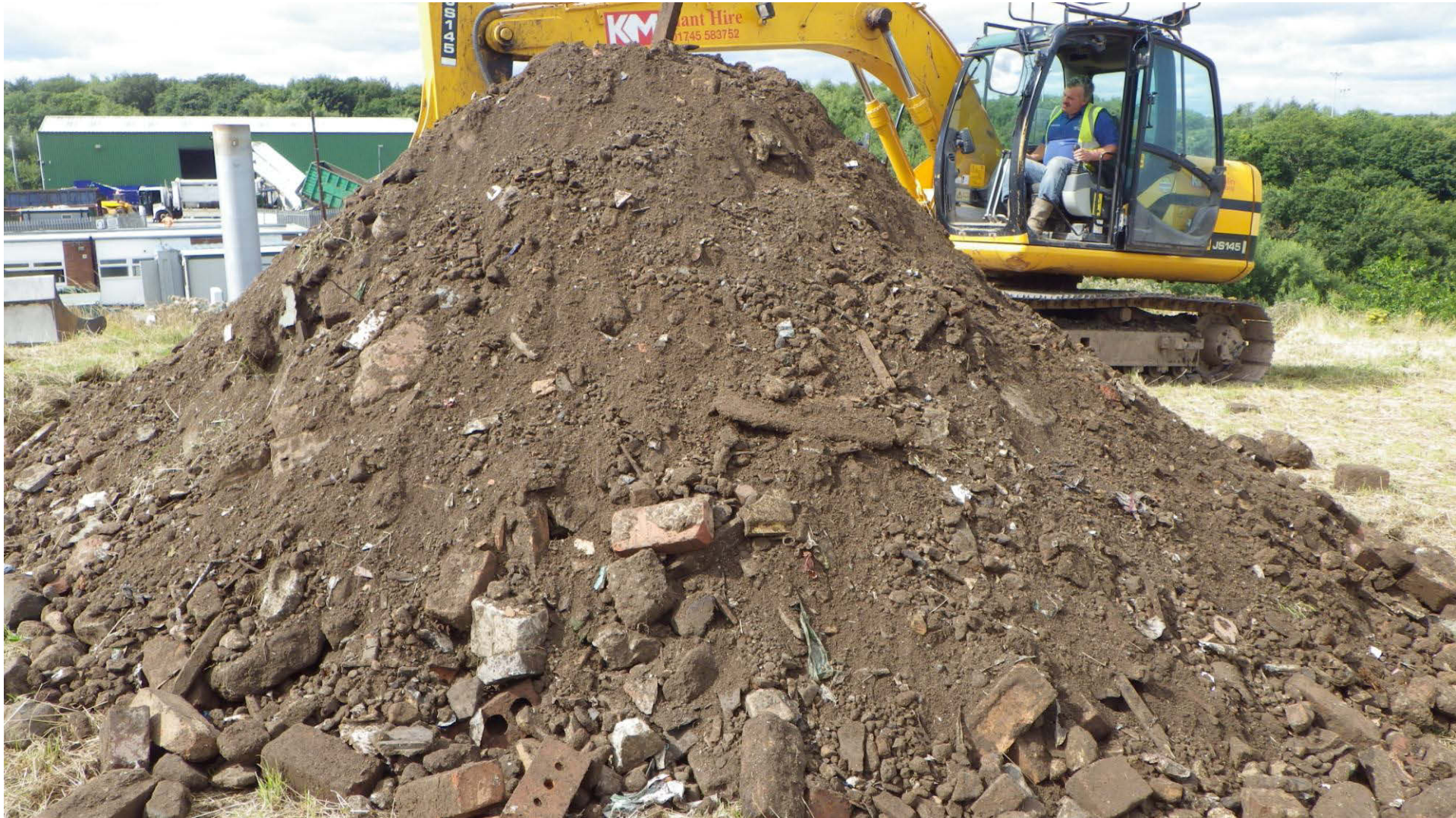
Taken on WPR stockpile on edge of Standard Landfill site, waste from trial pit 9 at 2m deep.
