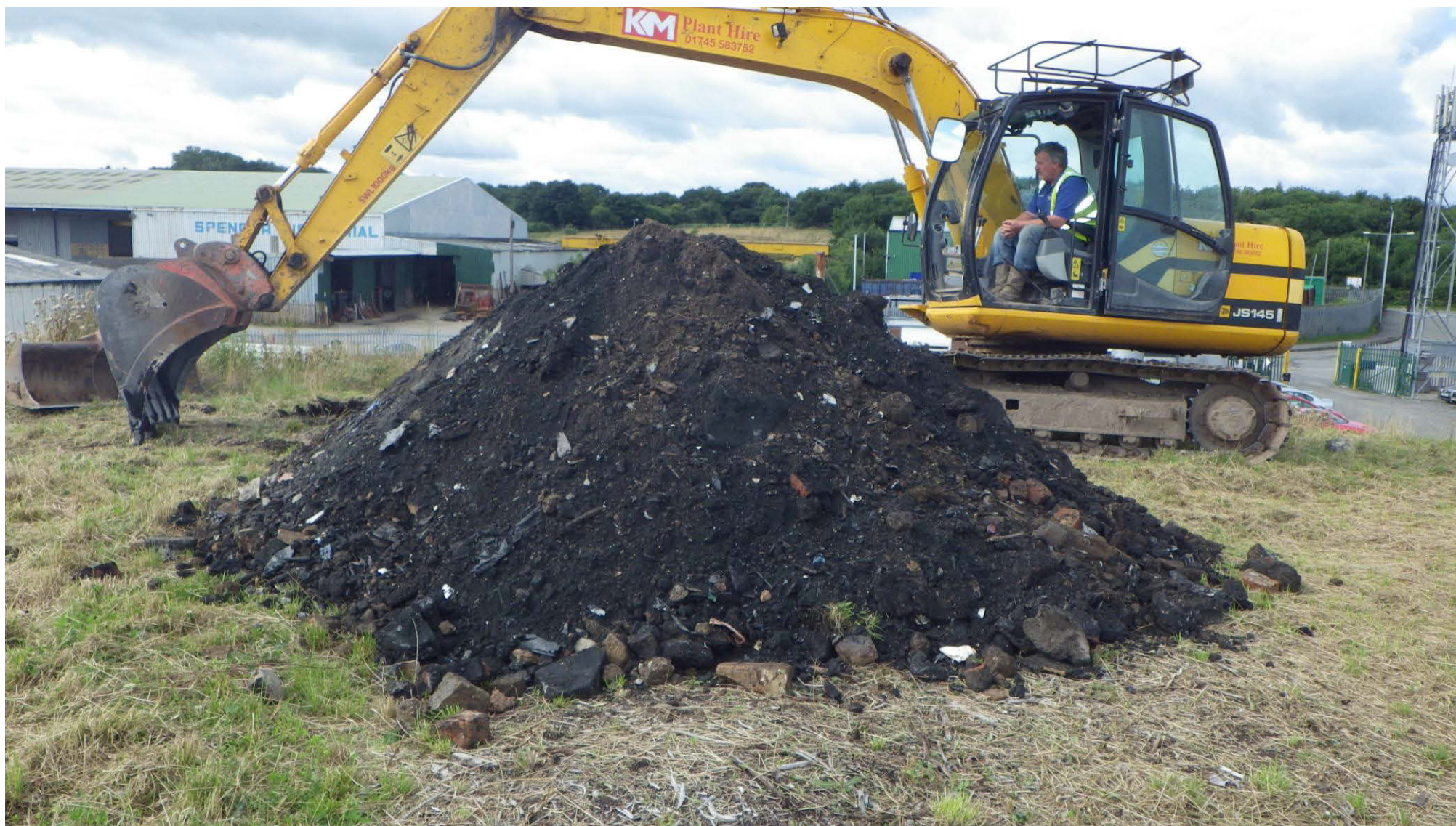
Taken on WPR stockpile on edge of Standard Landfill site, shows burnt waste from trial pit 10.
