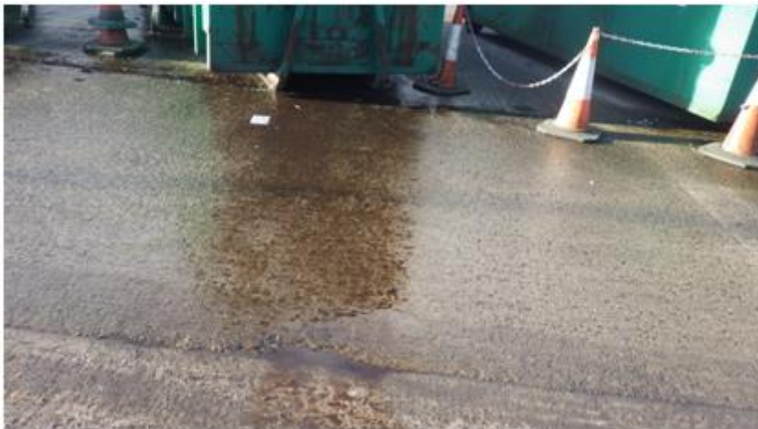
Leachate deriving from the storage of PAS100 compost
