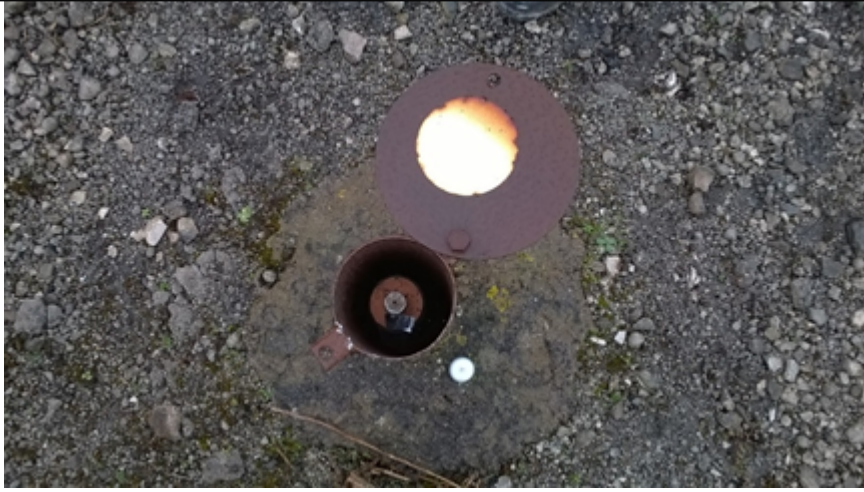
Figure 2 Gas Bore Hole BH#
