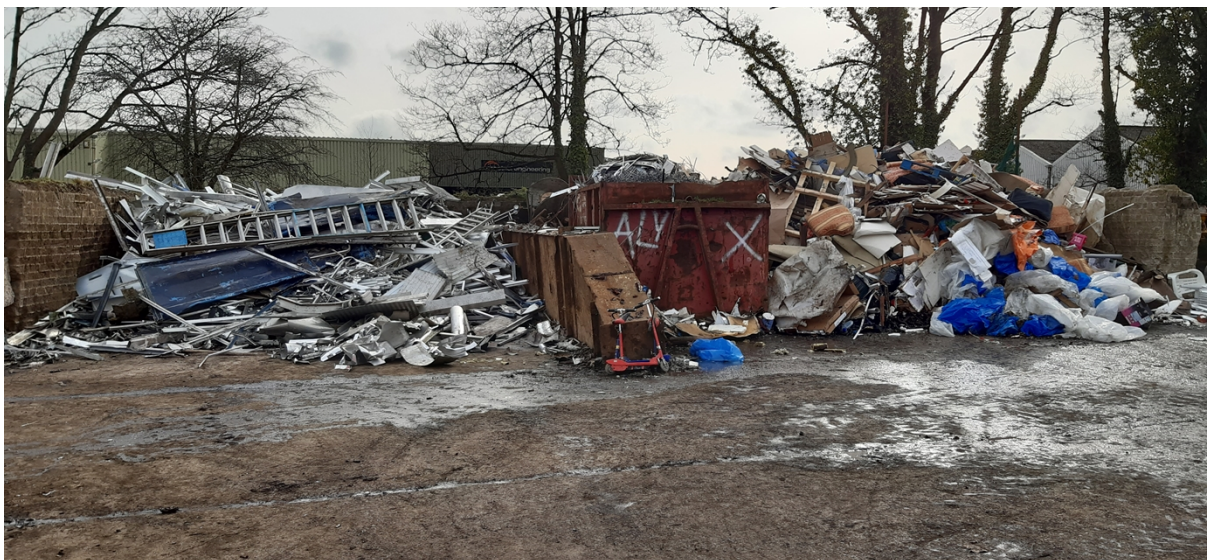
Photo 1 - General wastes stored in designated / segregated bays
