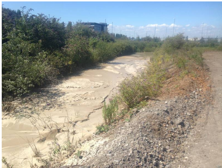
Plate 1. Leachate Collection Ditch at southwest corner of site
