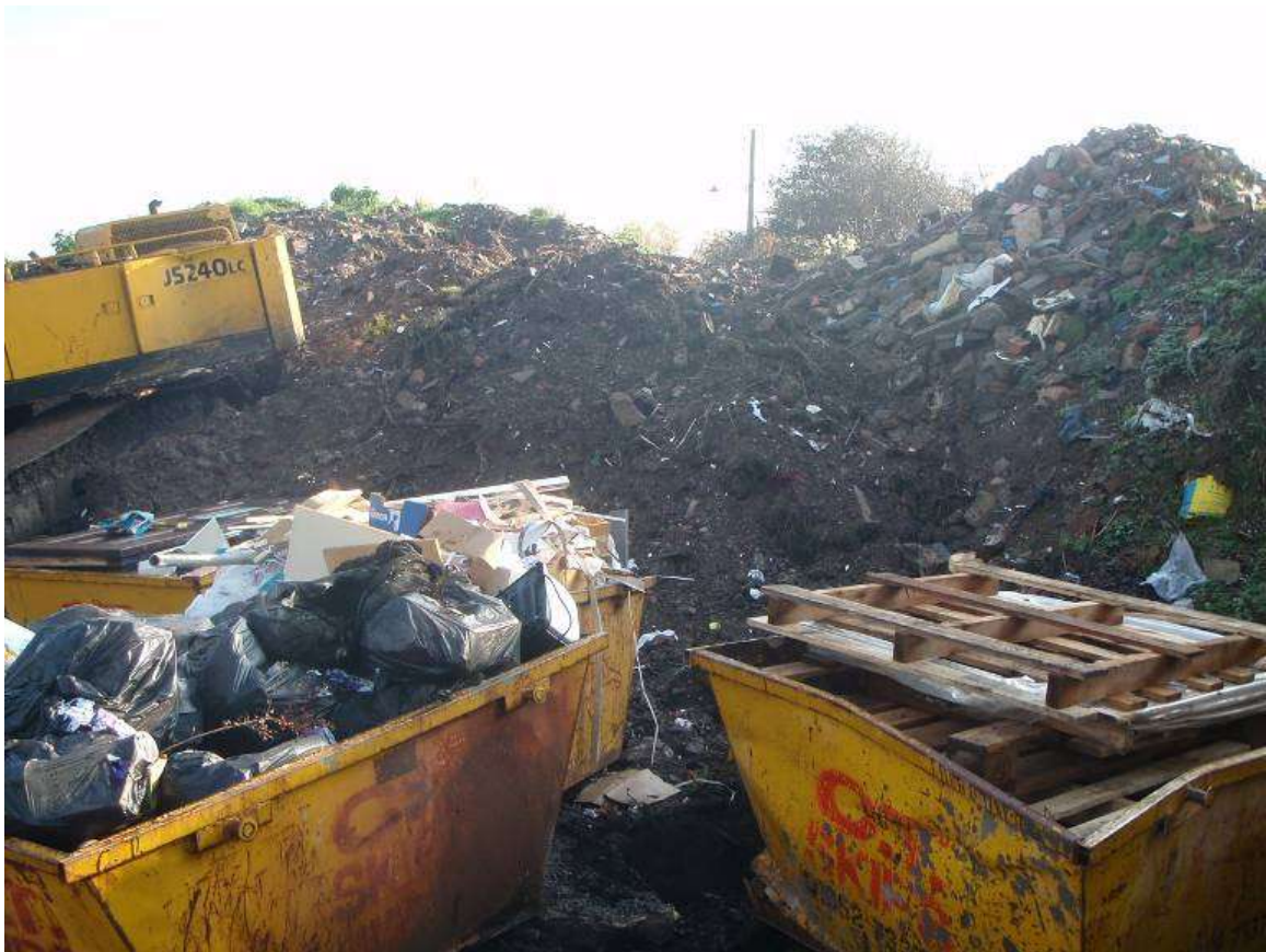
Photograph above shows general view of the site, contaminated soil waste behind skips
