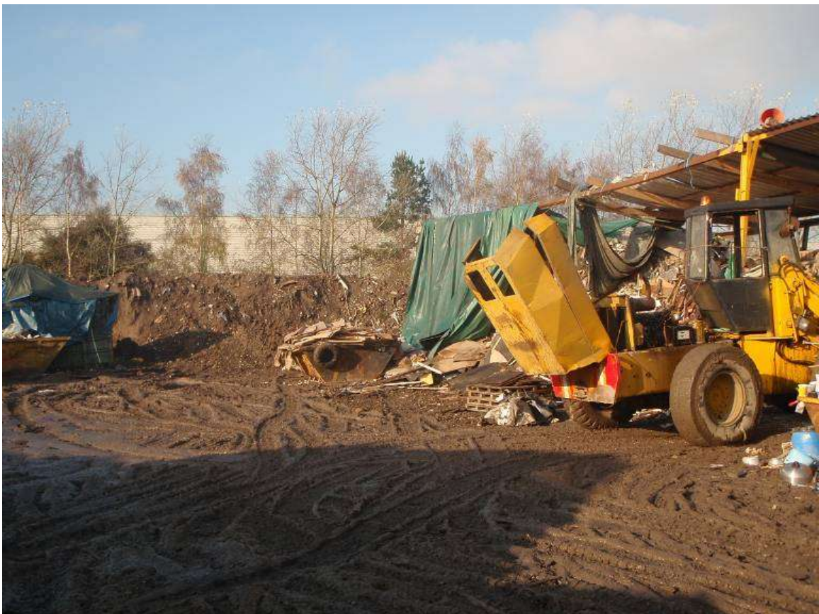
Photograph above shows general view of the site
