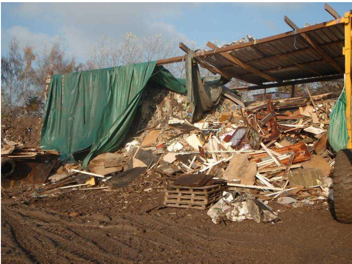
Photograph above shows waste storage building on site
