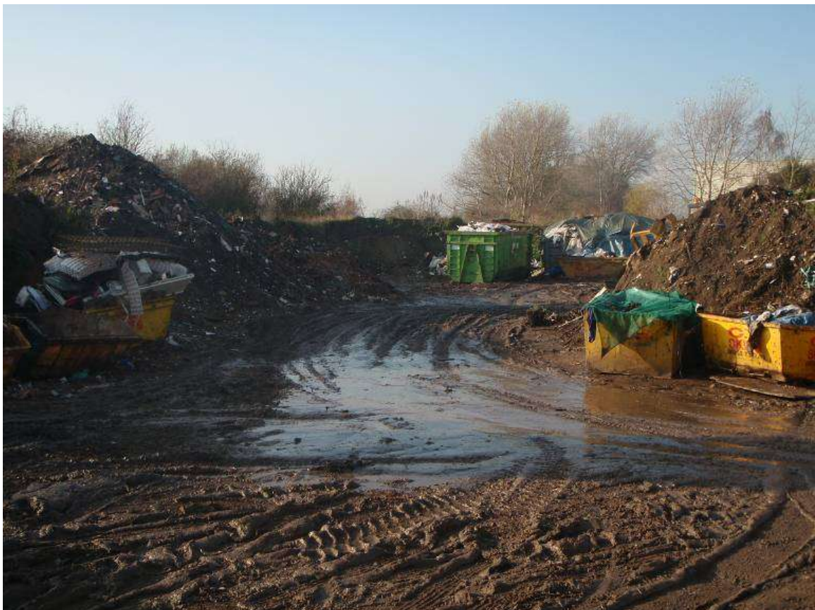
Photograph above shows mud and general view of the site
