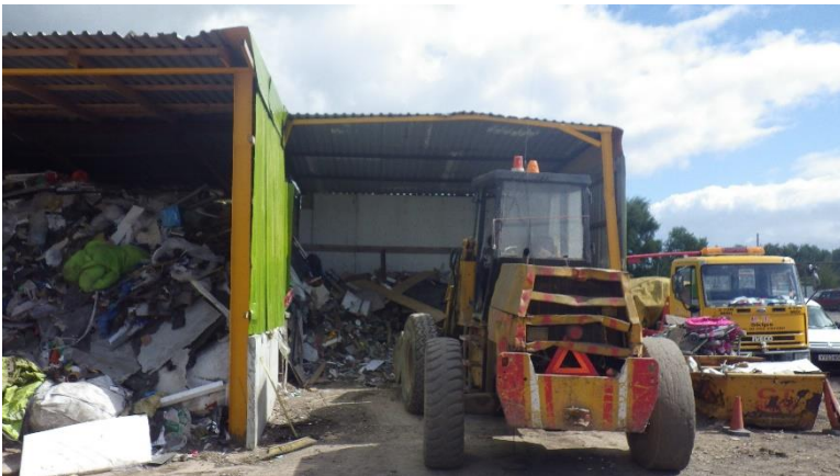
Sorting bay building to be extended
