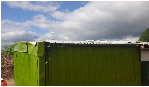
Sheeting to side of building and improvements to some of the back section
