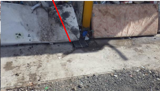
Concreted area in front of building and location of drain
