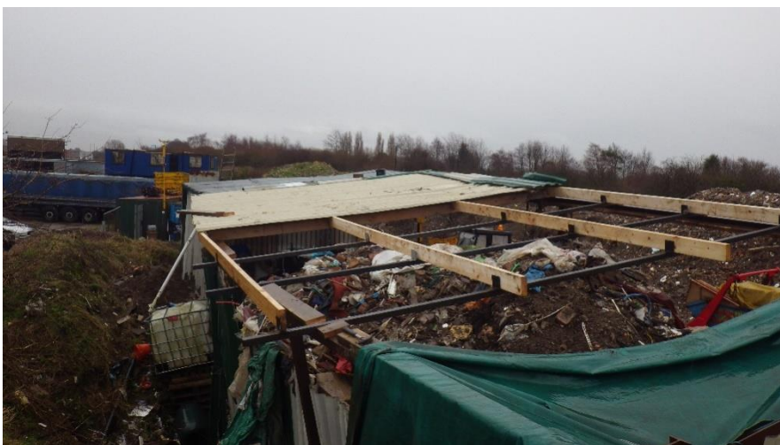
Repair on the roof has commenced on site.
