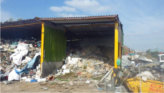
Building covering the sorting bay (closest to the main entrance gate) has been extended and is now in line with the storage bay.
