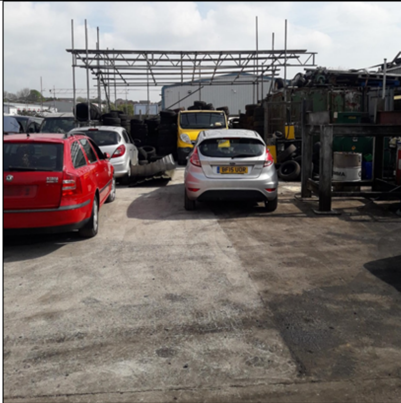
Picture 1 – showing newly concreted surface ready for the second depollution bay
