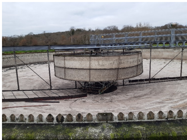
Photo 5: FST 3 drained for centre bearing repairs.
