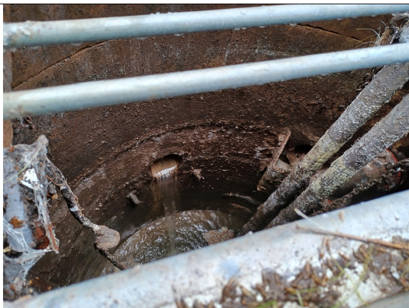
Photo 1 - Wet well showing incoming flows and screen
