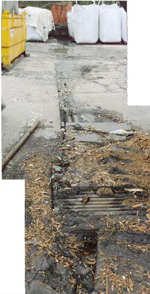
Figure 13. Linear cut-off drain and silt trap in front of the processing building in the southern yard area.
