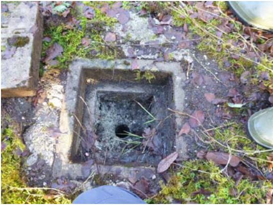
Photograph showing groundwater borehole. Casing flush with ground level.
