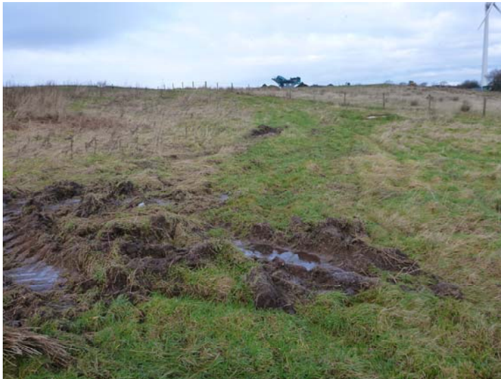
Photograph showing damage to the cap caused by vehicle. Approx. NGR:- SN4726317171
