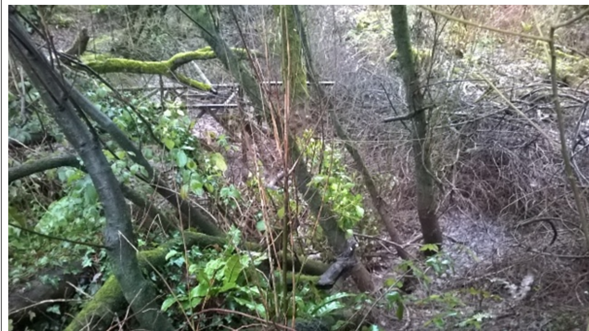
Photo 2 showing area of soakaway
