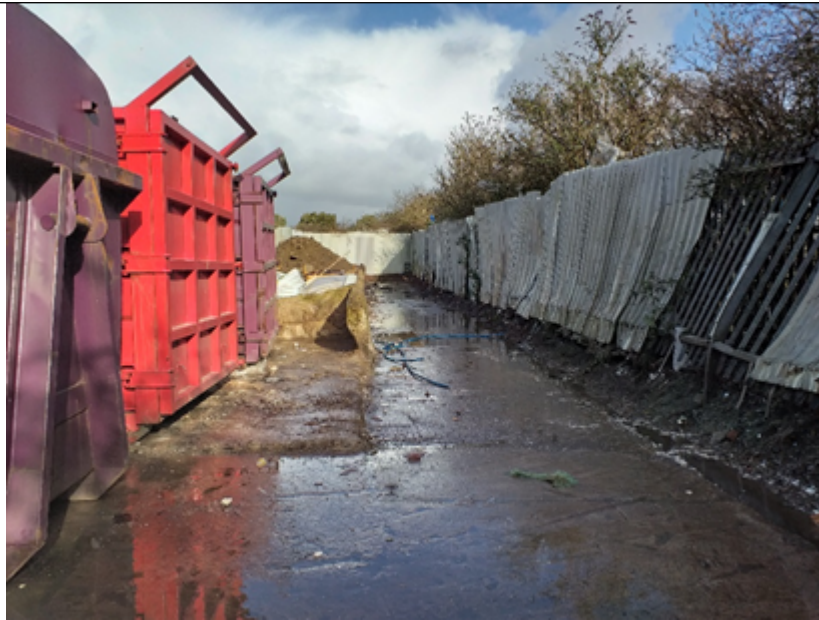
Image 1 – exposed ground on south-east edge of the sites perimeter
