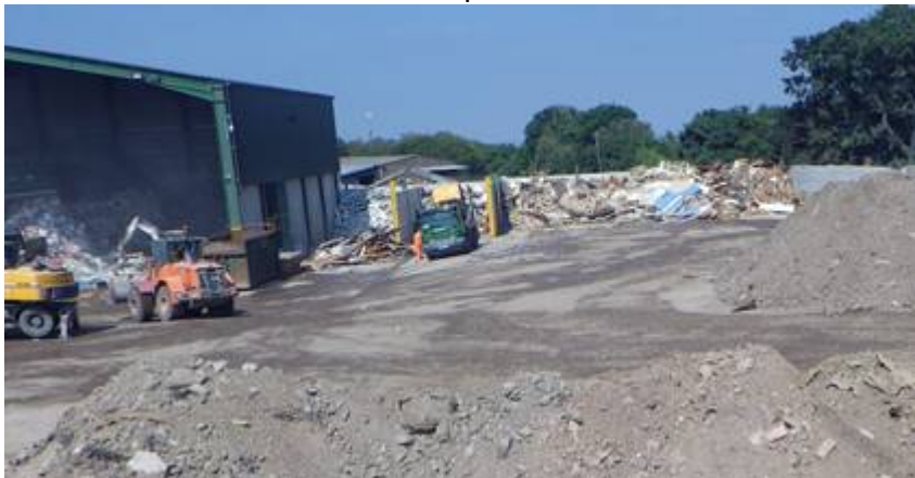
Photo 2 – Bay outside the new transfer building where mixed waste was being stored prior to treatment.
