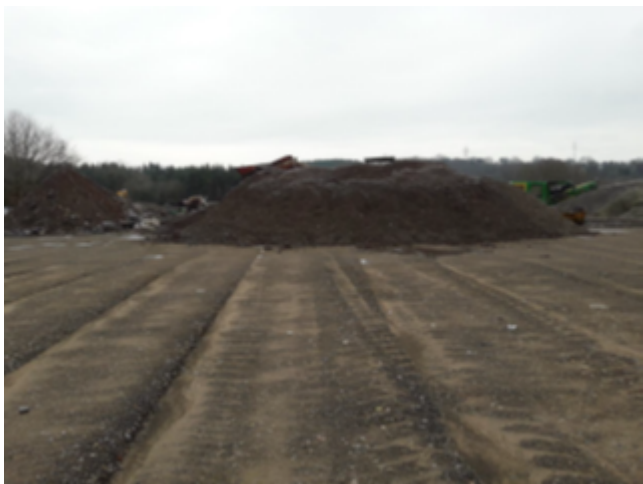
Image 2 – Evidence of waste being deposited on site rather than being recovered and exported, as well as evidence of levelling of other waste material on flattened surfaces.
