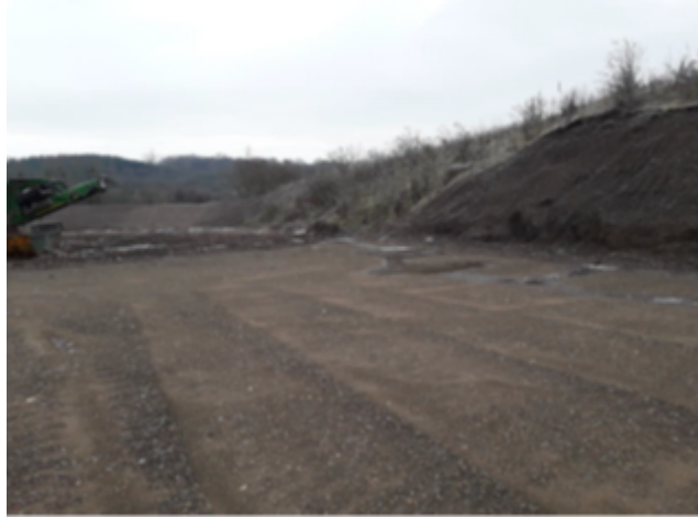
Image 3 – Further evidence of levelling on site.
