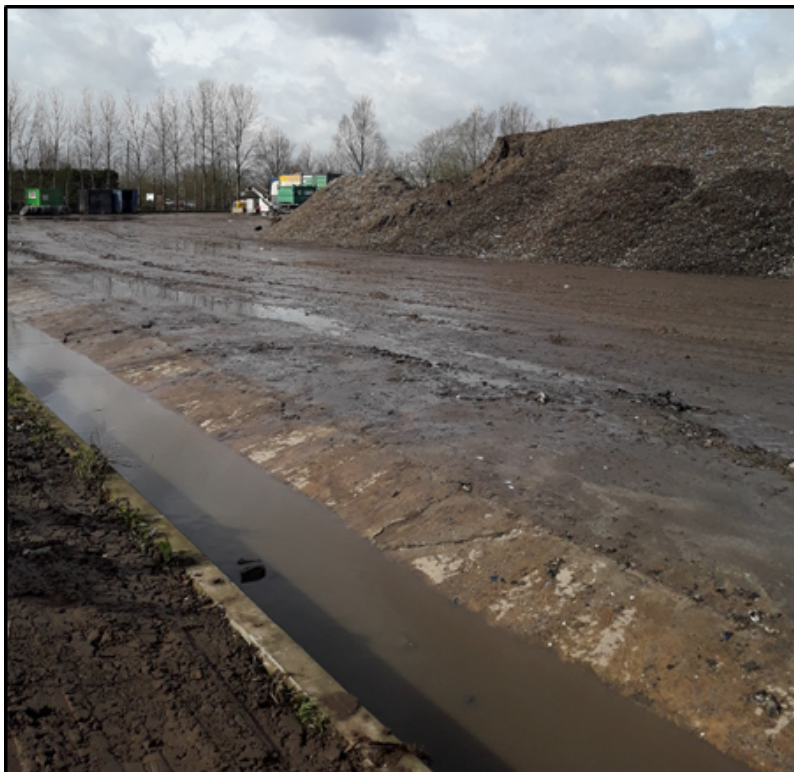
Picture 3 – showing the designated quarantine area in Field 1, taken on 14/03/19
