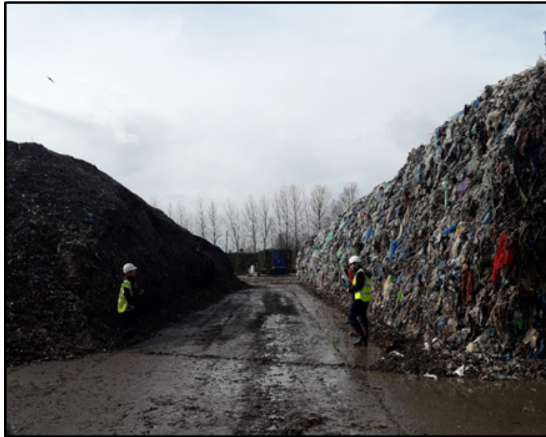
Picture 2 – showing an inadequate separation distance between Stockpile 2 and 12, taken on 14/03/19
