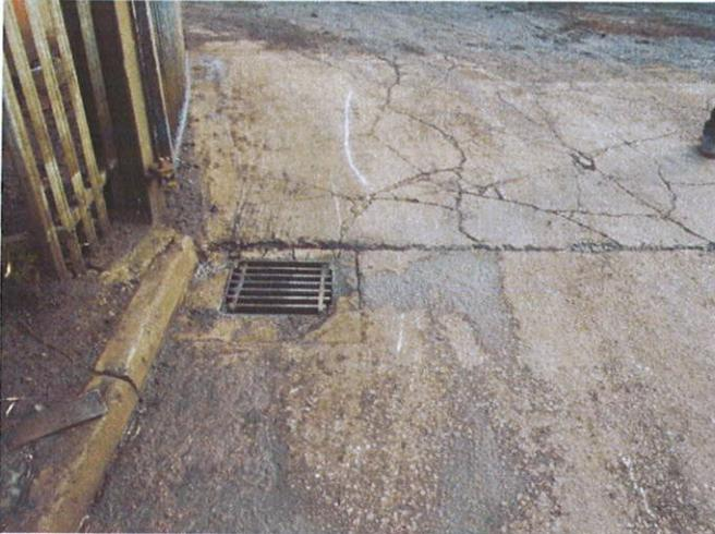
Large quantities of waste are stored on unmade ground. All waste must be stored on an impermeable surface\* with a sealed drainage system (*see definition below*).
