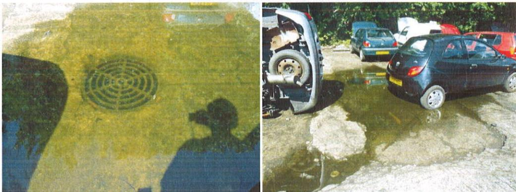
To become compliant with this condition the site must install a sealed drainage system with all operational areas (where waste is stored/treated) benefiting from impermeable surfaces.
