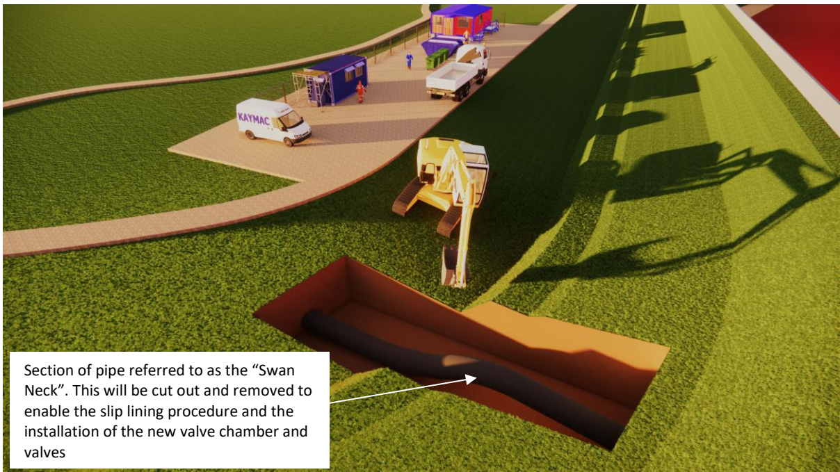
Illustration showing the approximate location of the excavation required to expose the existing pipe for replacement and for the construction of the valve chamber (the temporary excavation support system has been omitted for clarity)
