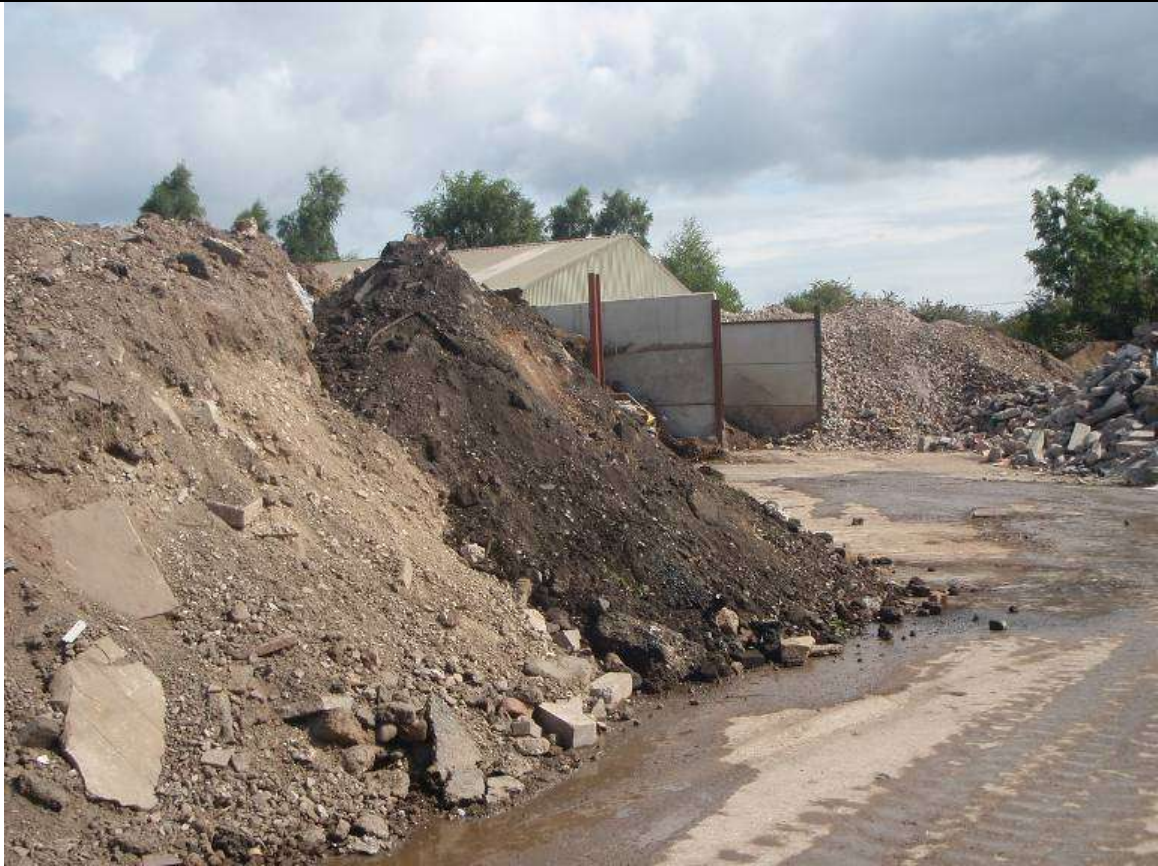
Photograph above shows storage of soil and aggregate material
