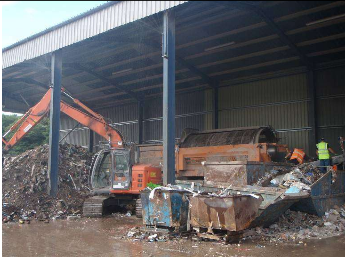
Photograph above shows the main waste building, with dust suppressing sprinklers visible in operation on the pillars.
