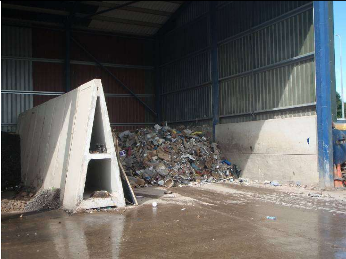
Photograph above shows a mixed construction and demolition waste bay within the main building
