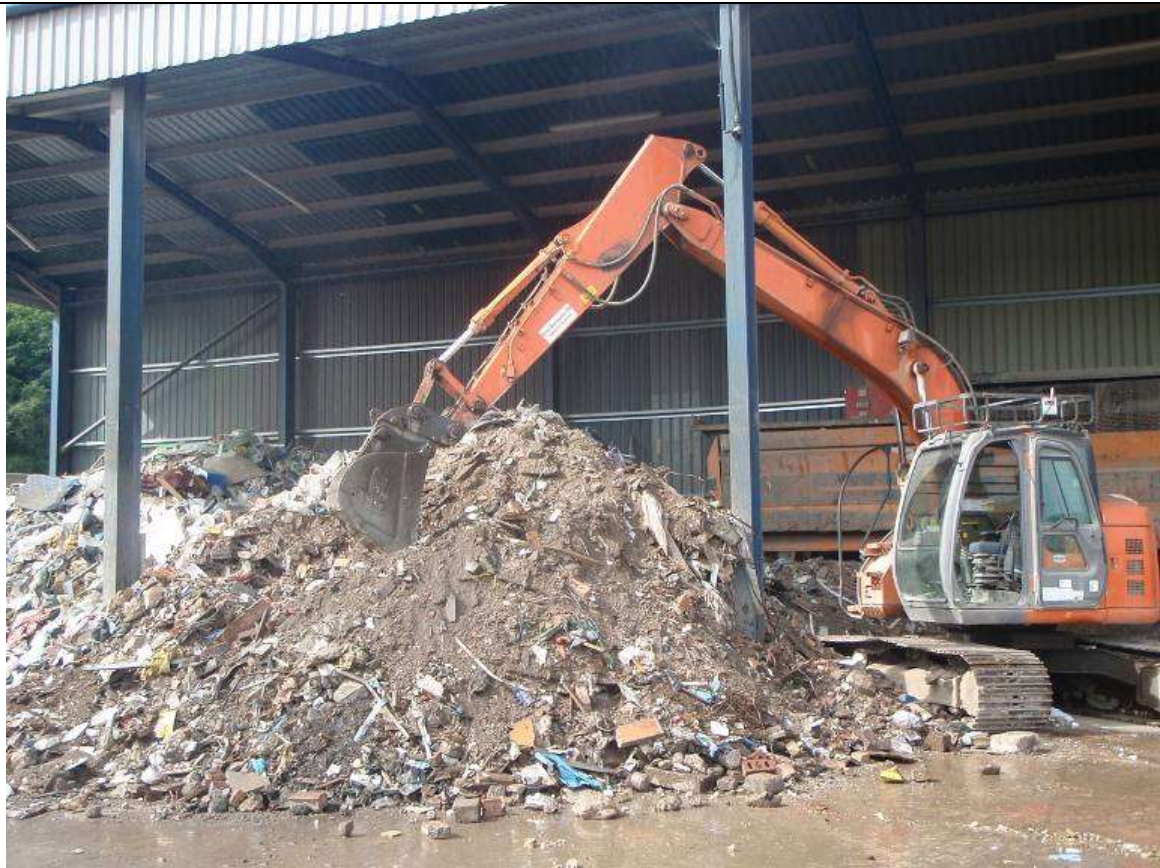
Photograph above shows the main waste sorting building
