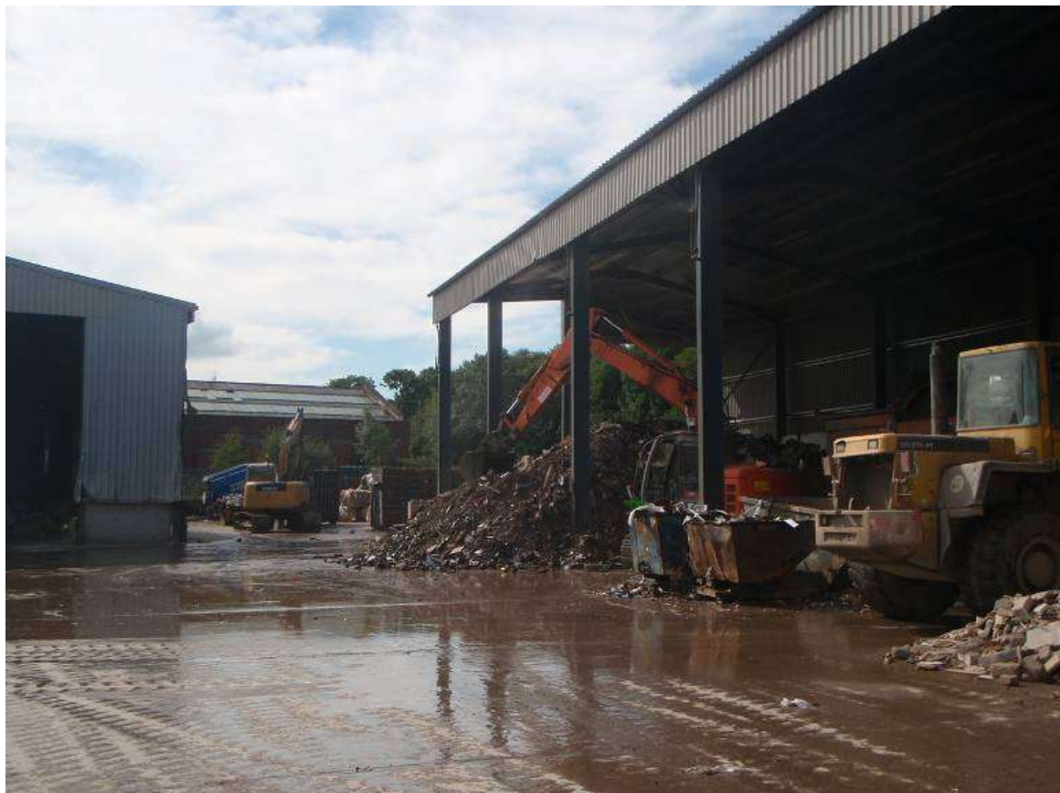
Photograph above shows the exterior of the main waste building.
