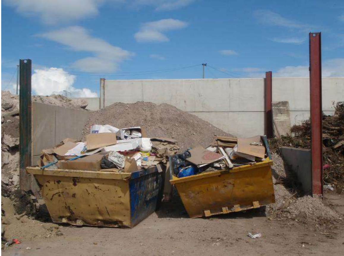
Photograph above shows some temporary skip storage in a waste bay
