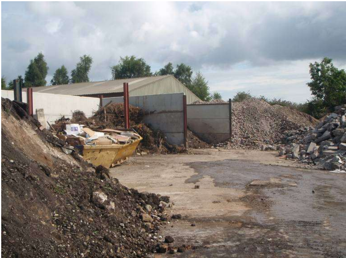
Photograph above shows a general view of the aggregate recycling area
